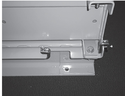
Figure 1 : Installation d'une attache-support
