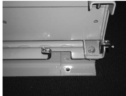
Figure 1: Beam Clamp Installation
