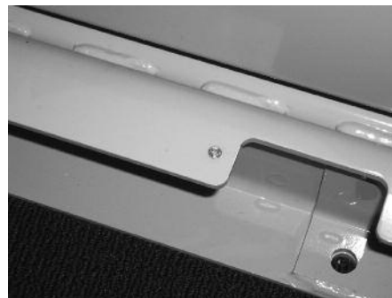
Figure 2: Adequate Paint Penetration
