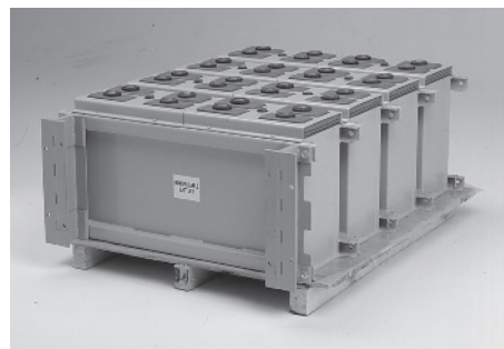
I-BEAM SUPPORT INSTALLED Figure 8
